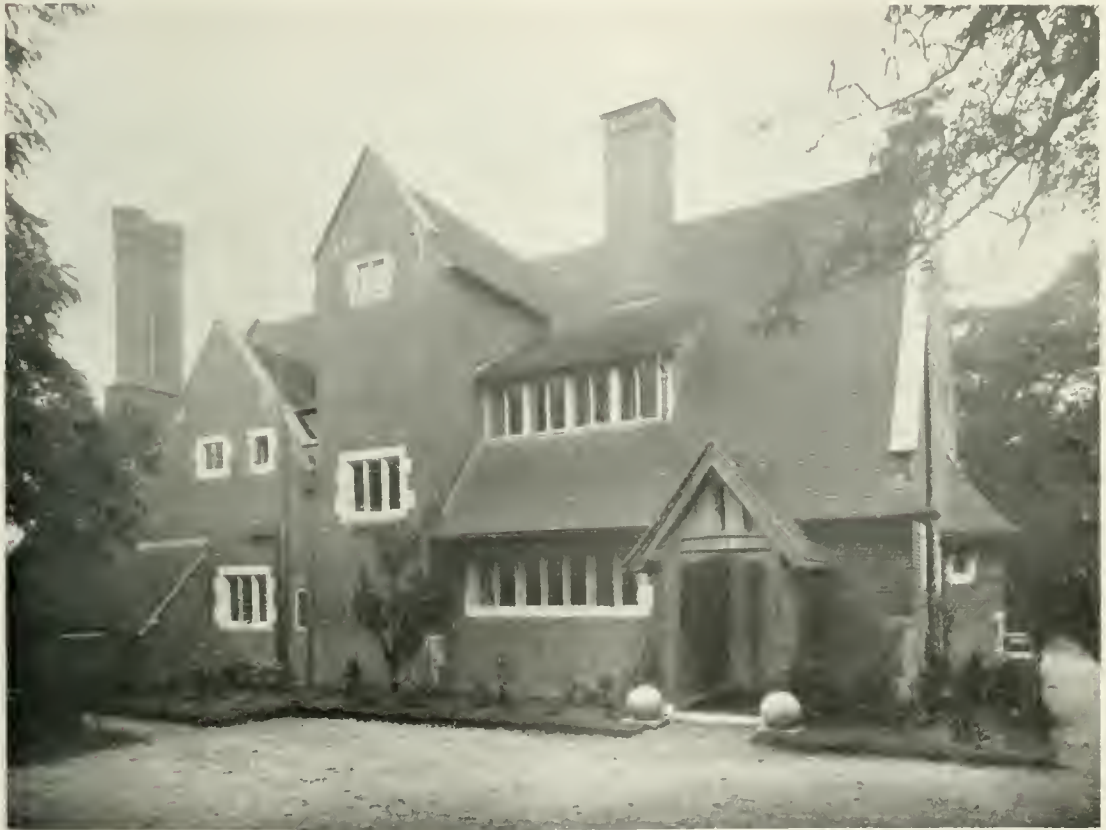
B15 THE GARDEN FRONT, WOODGATE, FOUR OAKS. IT IS ROOFED WITH DARK TILES AND BUILT OF MULTI-COLOURED THIN BRICKS
